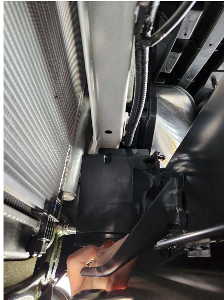
Figure 3: Installer removing the plastic deflector.
